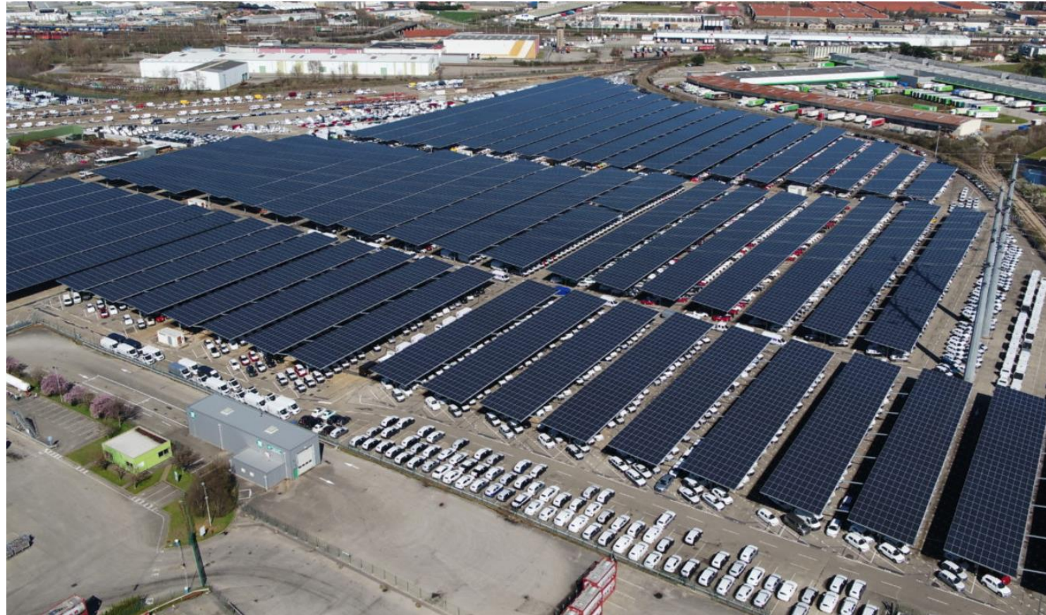
16 MW Corbas solar carport installed by Neoen, in France
